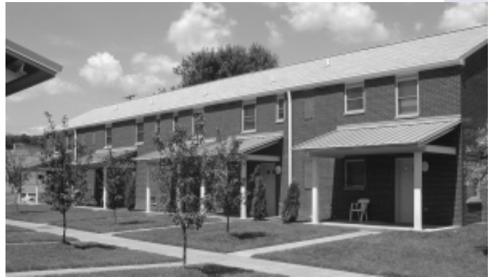
The same building AFTER undergoing modernization
