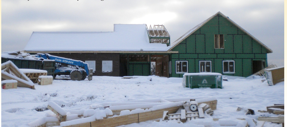
February 2015 - Community Building Construction
