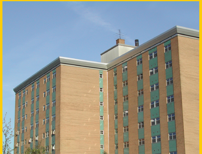
General Braddock Tower new windows roof & roof cornice
